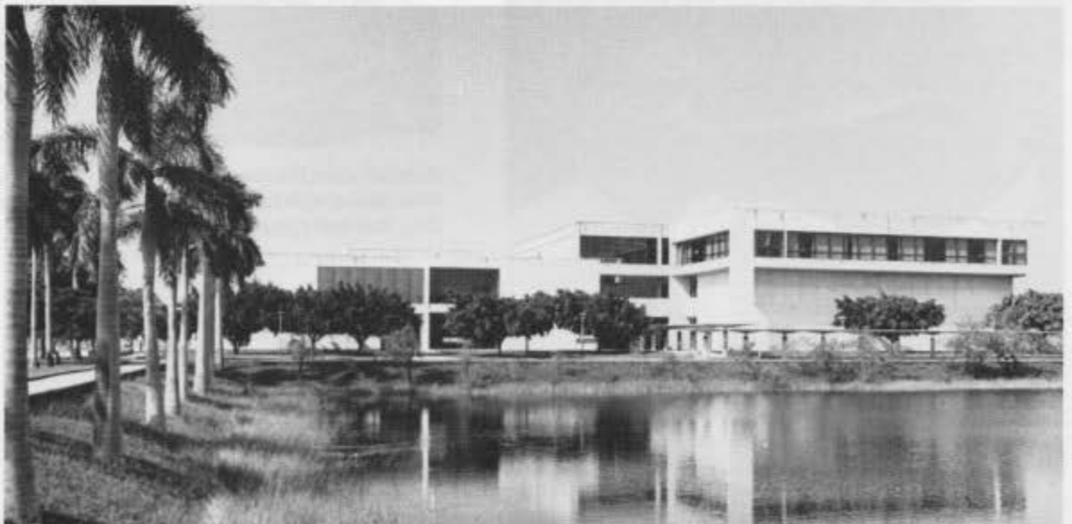
Criminal Justice Building and Garth Reeves Classroom Building on the North Campus.
