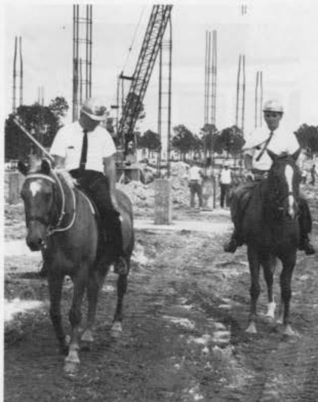
The construction area was so large and so rough that contractors and overseers took to horseback to keep track of daily activities. Miami-Dade construction supervisors George Crew and Don Bulat.
