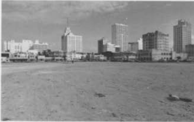
The site for a new downtown campus was cleared in February 1971.
