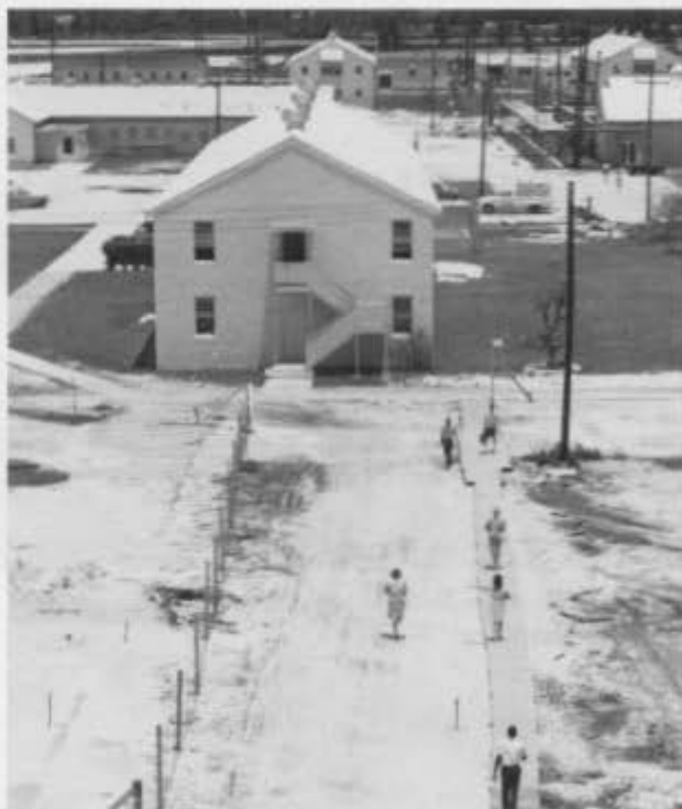
Students and construction crews share space as the old Masters Field becomes a campus.
